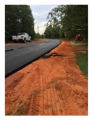
SoilBinder<sup>®</sup> provides a sturdy base for any type of wearing surface: Chip & Seal, HMA, Concrete, seal coating, etc.
