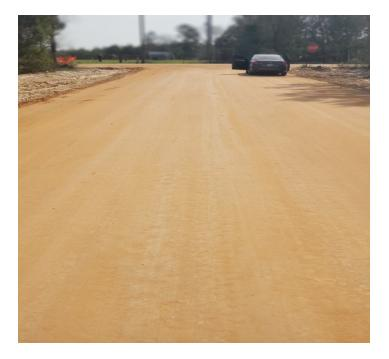
Hydrating the base is recommended when working under extremely hot weather or with sandy soils.
